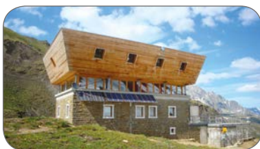
Capanna Corno Gries
